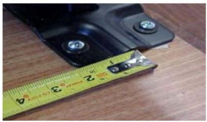
Put the legs (legs are called "standards" in the seating business) in an upright position where you would like them to go, from the center of one standard to center of the other standard should be exactly 22 inches apart.
